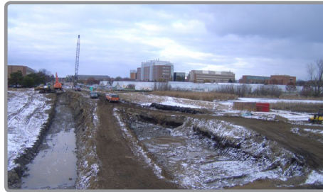
Wintertime construction in Michigan. Image: MSU IPF (via Flickr CC)
