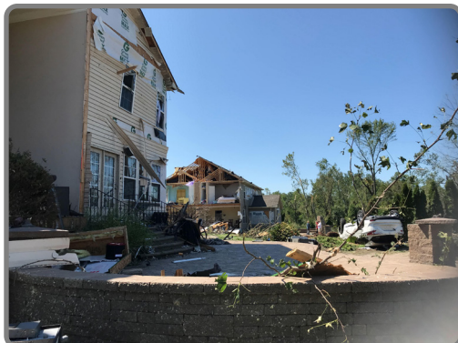
Damage from an EF-3 tornado in Mullica Hill, NJ. Credit: NWS Philadelphia
