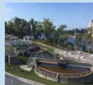
Cape Fear Public Utility Authority, North Carolina
