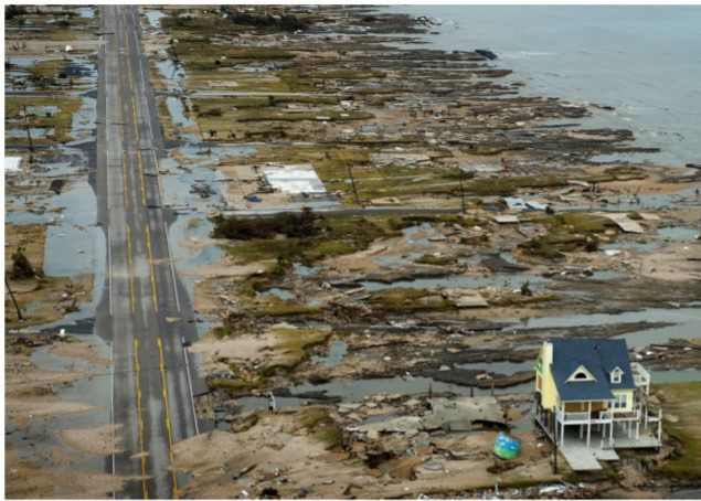
BOLIVAR PENINSULA IN TEXAS AFTER HURRICANE IKE (2008)
