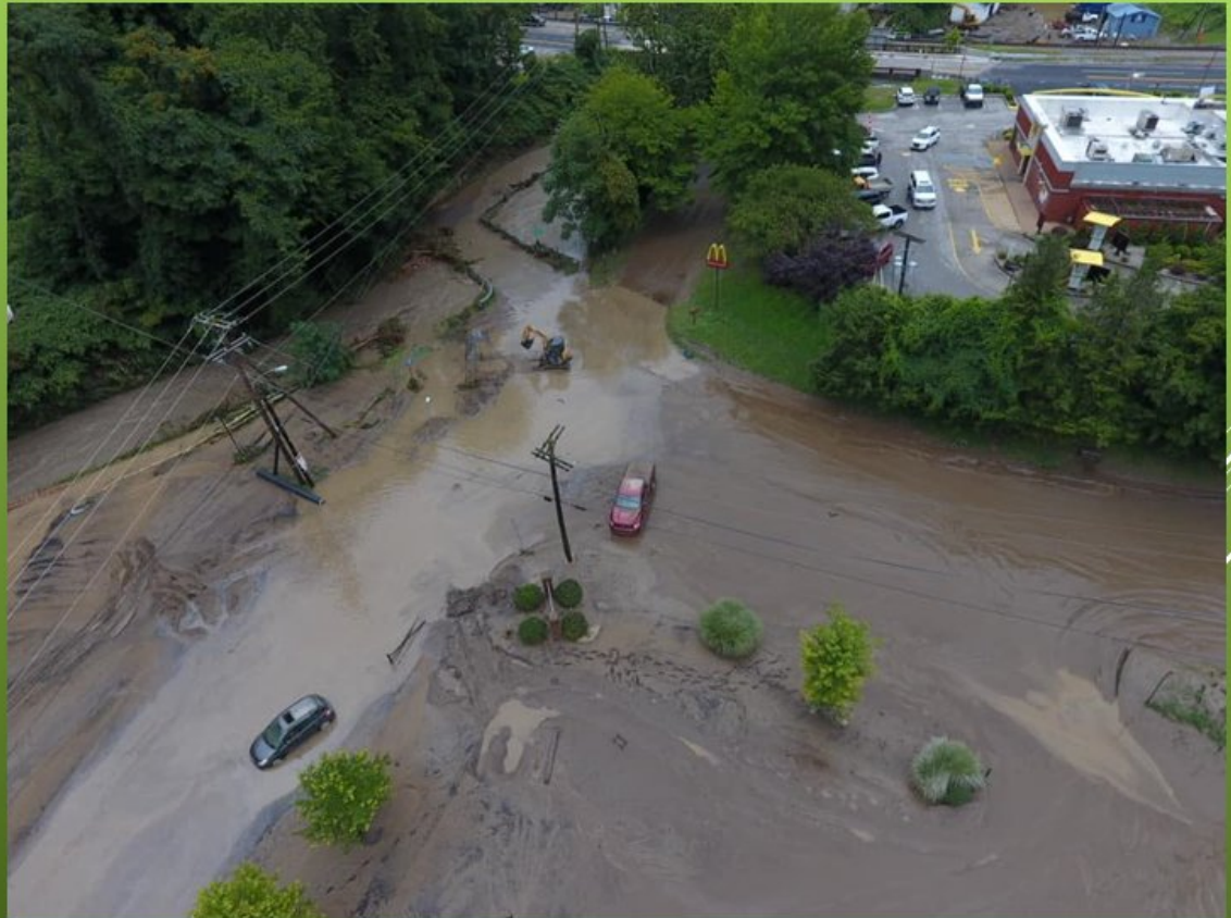
Flooding & Aftermath in Smithers, WV. Credit Fayette Cty Sheriff's Office
